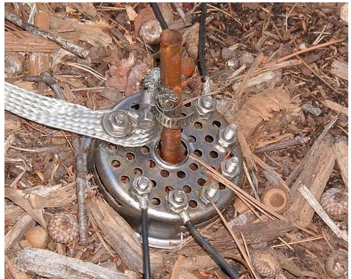
In my installation, each screw is fastened to the strainer with a compression lockwasher and nut. Then the radial lugs are placed over the nut and secured by a second nut. To prevent "galling" or seizing up of the stainless hardware, I placed Noalox grease on the screw threads. I also placed some grease on the flat surfaces of the lugs. Home Depot and Lowe's carry Noalox in the electrical section.
