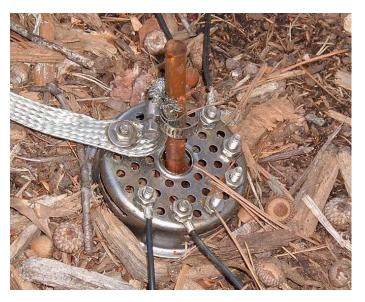
In my installation, each screw is fastened to the strainer with a compression lockwasher and nut. Then the radial lugs are placed over the nut and secured by a second nut. To prevent "galling" or seizing up of the stainless hardware, I placed Noalox grease on the screw threads. I also placed some grease on the flat surfaces of the lugs. Home Depot and Lowe's carry Noalox in the electrical section.
