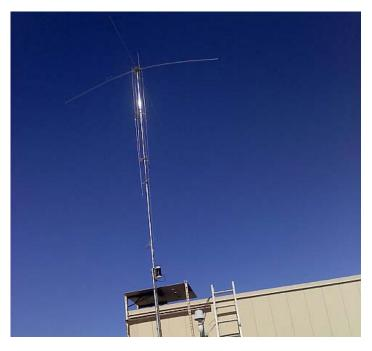
The weather was nice and not too windy for the work. While Bob and Ross ran coax between penthouse #6 and #4 using some Dacron line, the rest assembled the various antenna sections together as well as assembling the counterpoise system cables. Some of the grounding lugs had to be replaced as the supplied ones had no chance of fitting around a 1/4" bolt. Also, we had to solder the cable used for the counterpoise.
