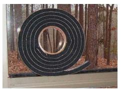
With this arrangement, air infiltration is minimal and bug infiltration is zilch. If you live in an area where it's really cold in the winter, you may want to better insulate that upper gap. But for the temperate climate of my upstate South Carolina QTH, I think the foam is sufficient.
