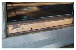
Since the window is partially open, you now have a gap between the glass in the lower sash and the frame of the upper sash (or the fixed frame of a single-hung window). Use the foam insulation to plug this gap, making sure you also plug any side gaps between the sash and the frame track. The actual strip of installed insulation is partly visible along the upper edge of the sash. I left the remnant of the insulation roll in the picture, resting on the sash, so you can see what the product is.
